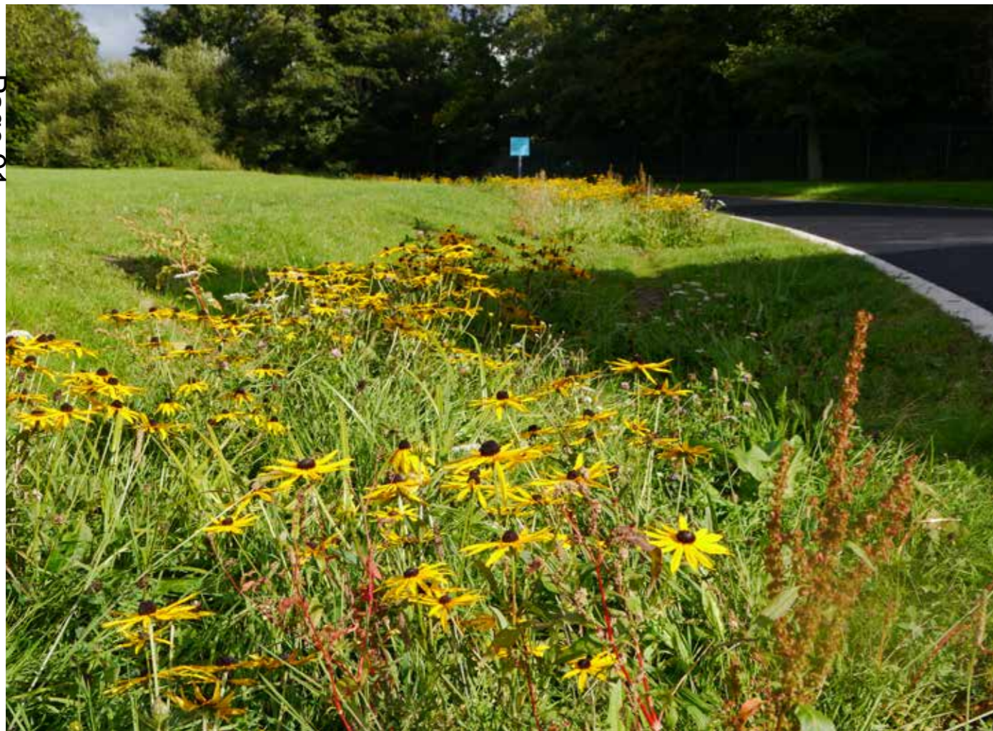
The final swale at Bewdley School is a colourful outfall into the existing watercourse.
