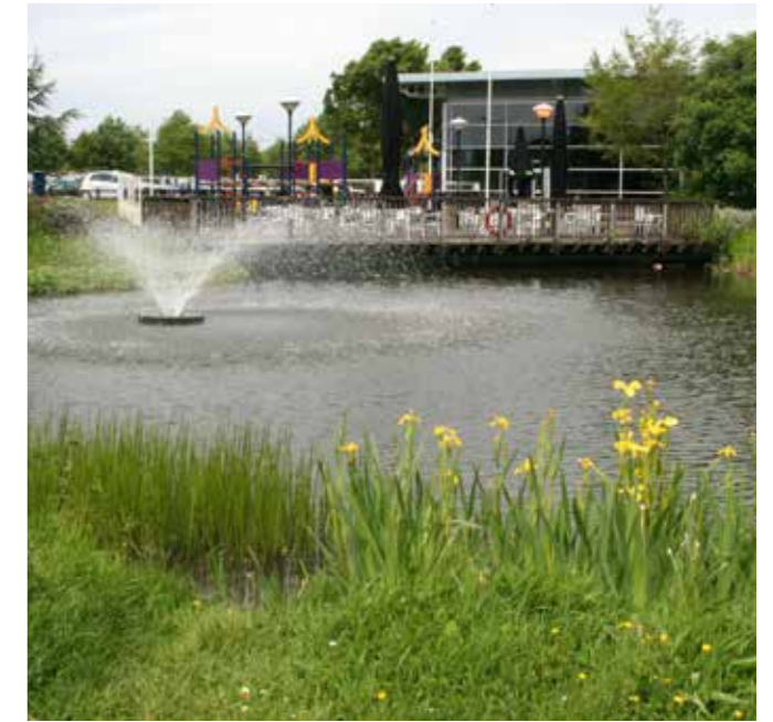
Hopwood Park MSA M42. Wooden terrace and balustrade with wet bench and planted aquatic bench protection to open water.
