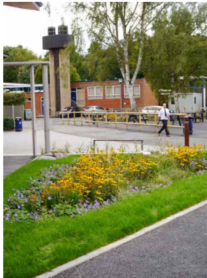
Longer SuDS grass as a filter strip between paved surfaces and a rain garden.
